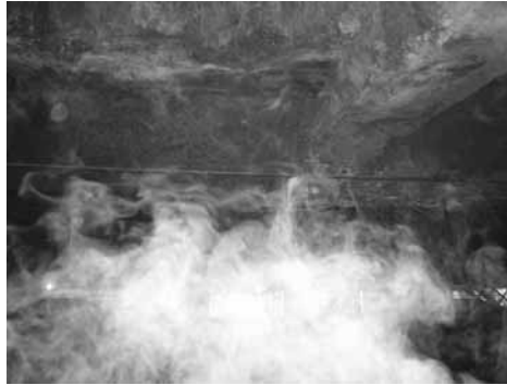
Fig. 1. Concrete structures exposed to the gases generated in water quenching of semicoke.
