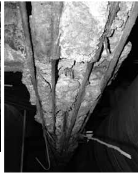
Fig. 3. Bottom view of a joist fragment carrying generator on the 2nd floor.
