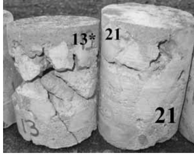
Fig. 6. Concrete cores 13* and 21 after drilling from columns.
